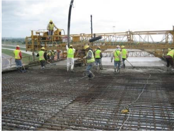
(b) Concrete being Placed and Vibrated
