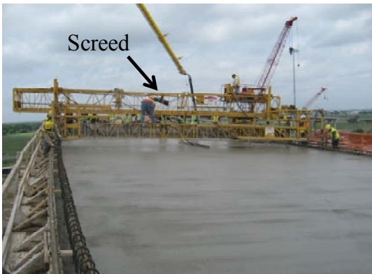
(a) Screed Leveling Concrete
