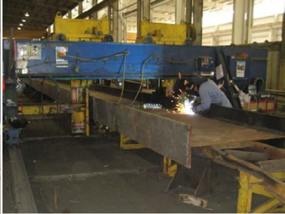
(b) Tack Welding of Flanges to Web
