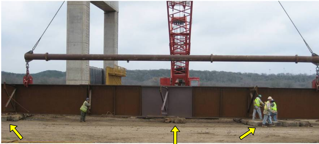
Figure 2.14: Large Wooden Support Timbers
