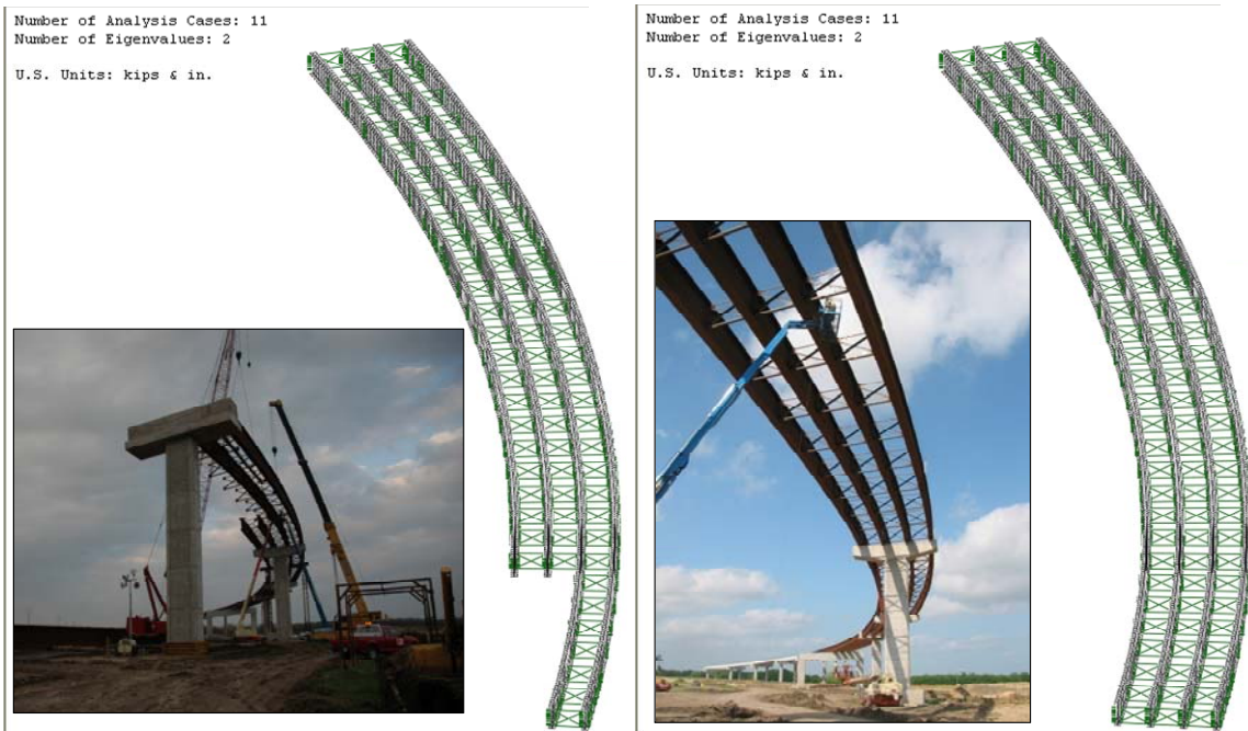
Figure 4.11: Bridge Erection Sequence with Associated UT Bridge Model
