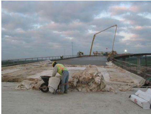
(d) Burlap Sacks Placed on Deck
