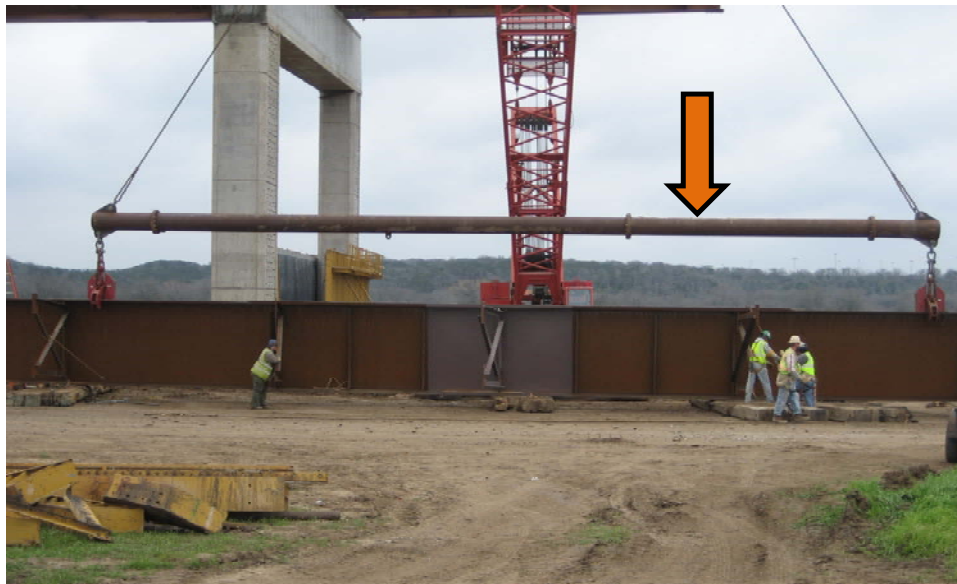
Figure 3.8: Spreader Bar used by a Single Crane Lifting a Girder
