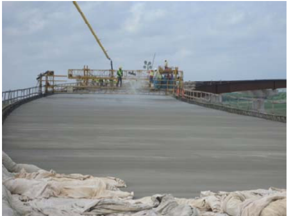
(c) Curing Compound Added to the Deck
