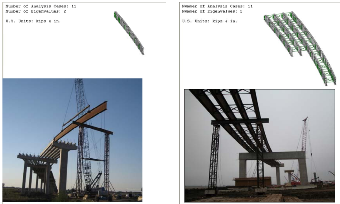
Figure 4.9: Bridge Erection Sequence with Associated UT Bridge Model
