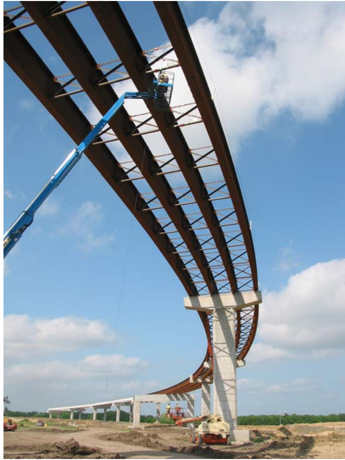
Figure 1.4: Curved I-girder Direct Connector Bridge in Austin, Texas during Construction
