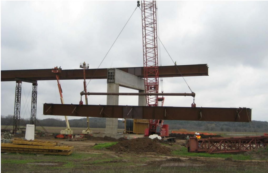
Figure 3.2: Lifting of a Horizontally Curved Steel I-Girder with 1 Crane & 2 Lift Clamps
