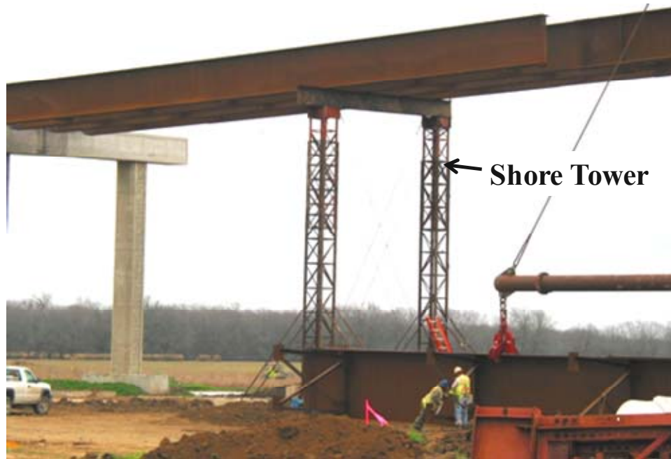
Figure 1.14: Temporary Support used for Stability Girder and Controlling Deflections
