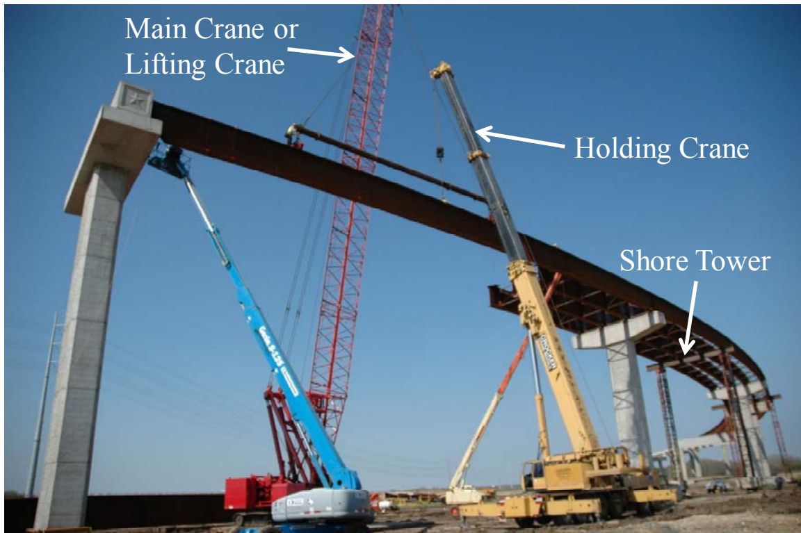
Figure 1.13: Curved I-girder Bridge during Erection
