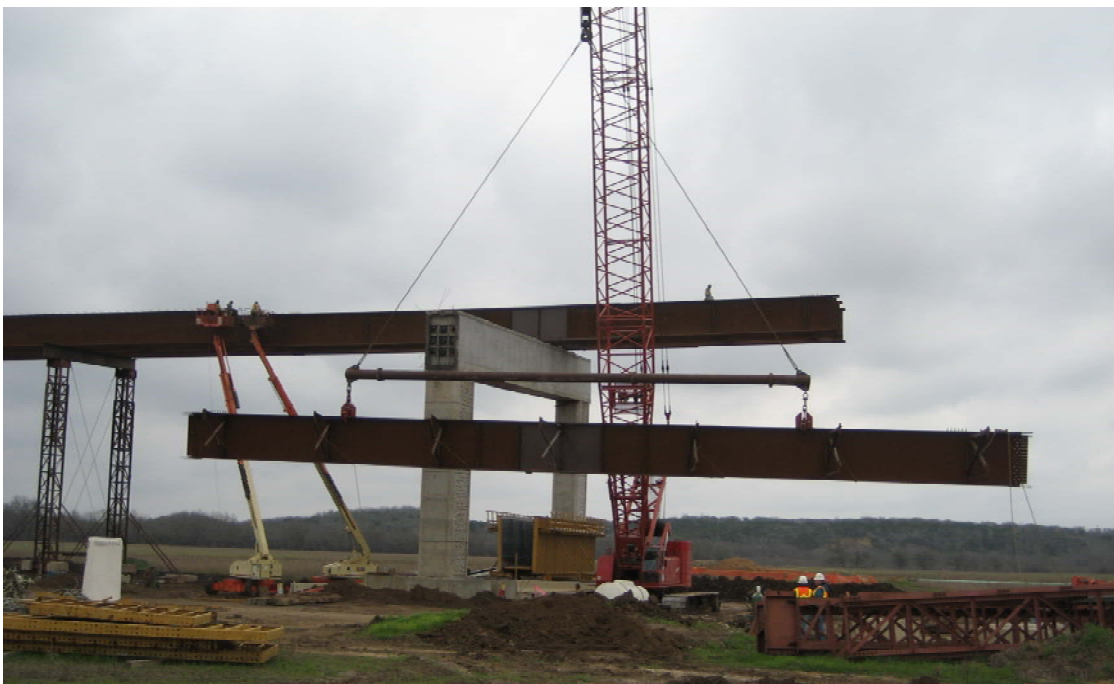
Figure 3.27: Lifting of a Horizontally Curved Steel I-Girder with 1 Crane & 2 Lift Clamps
