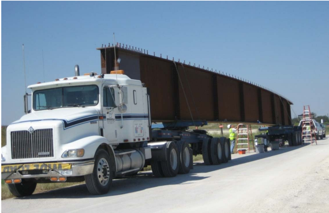
Figure 1.8: I-girder Transported by Truck to the Jobsite
