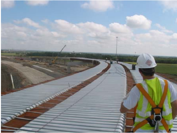
(a) Permanent Metal Deck Forms
