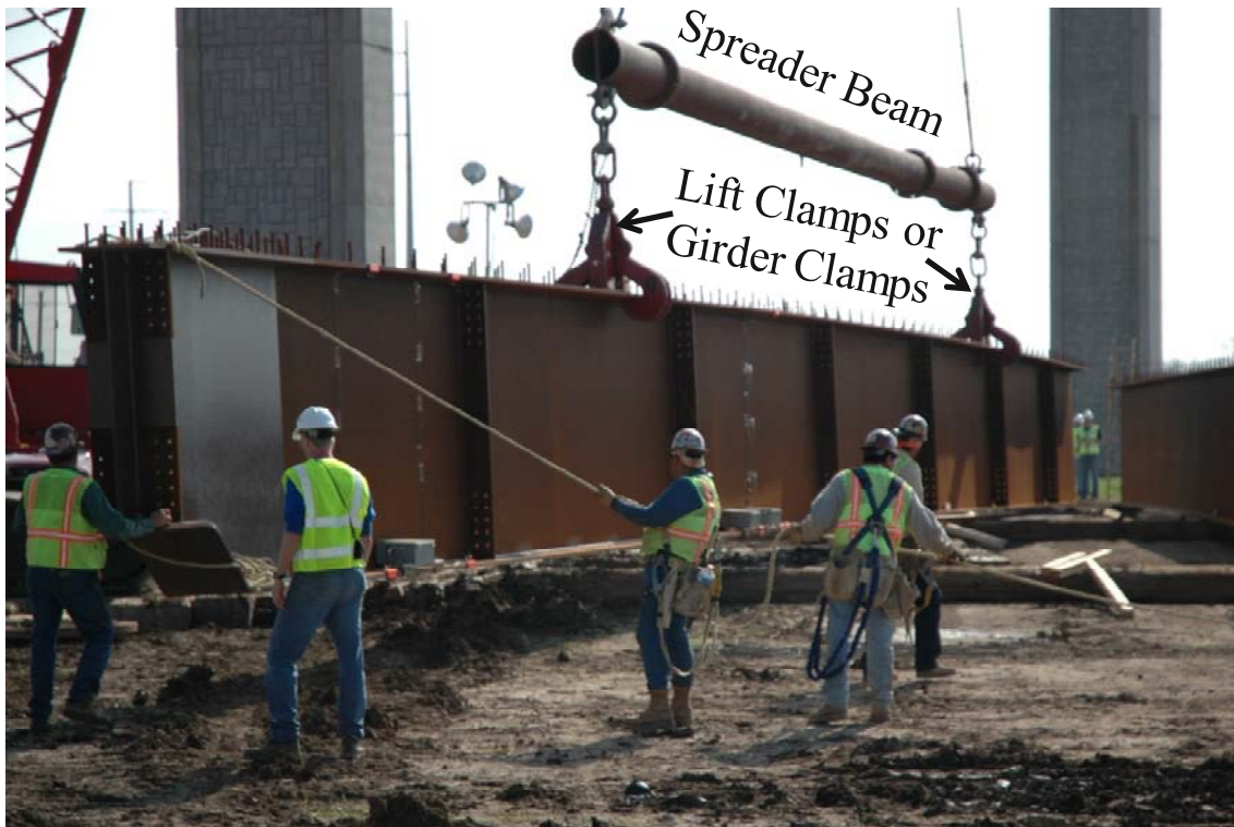
Figure 1.9: Curved I-girder Lifted with a Single Crane using a Spreader Beam
