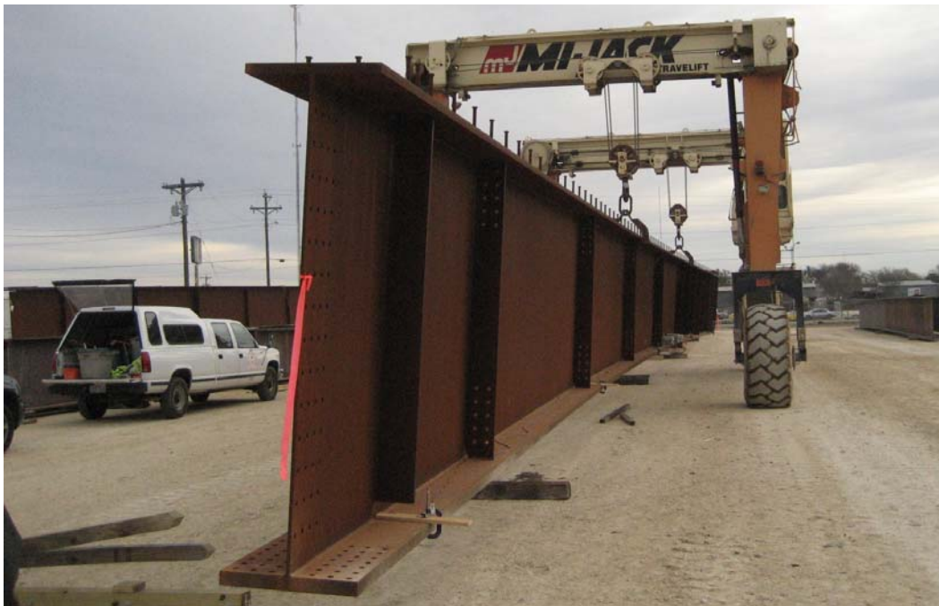
Figure 2.24: Actual I-girder Lifted during Field Test
