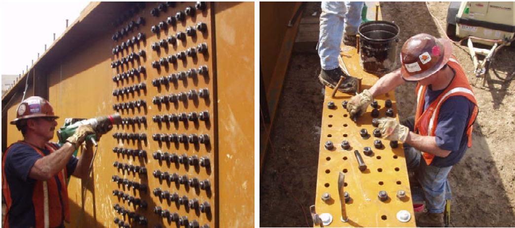
(a) Bolting Web Splice Plates
