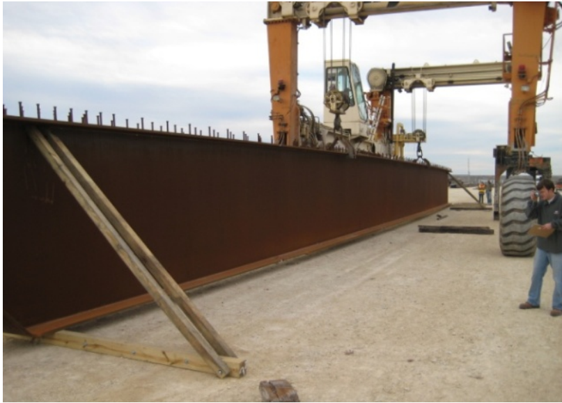
Figure 2.16: Fabricated Wood Supports for Girder Lift
